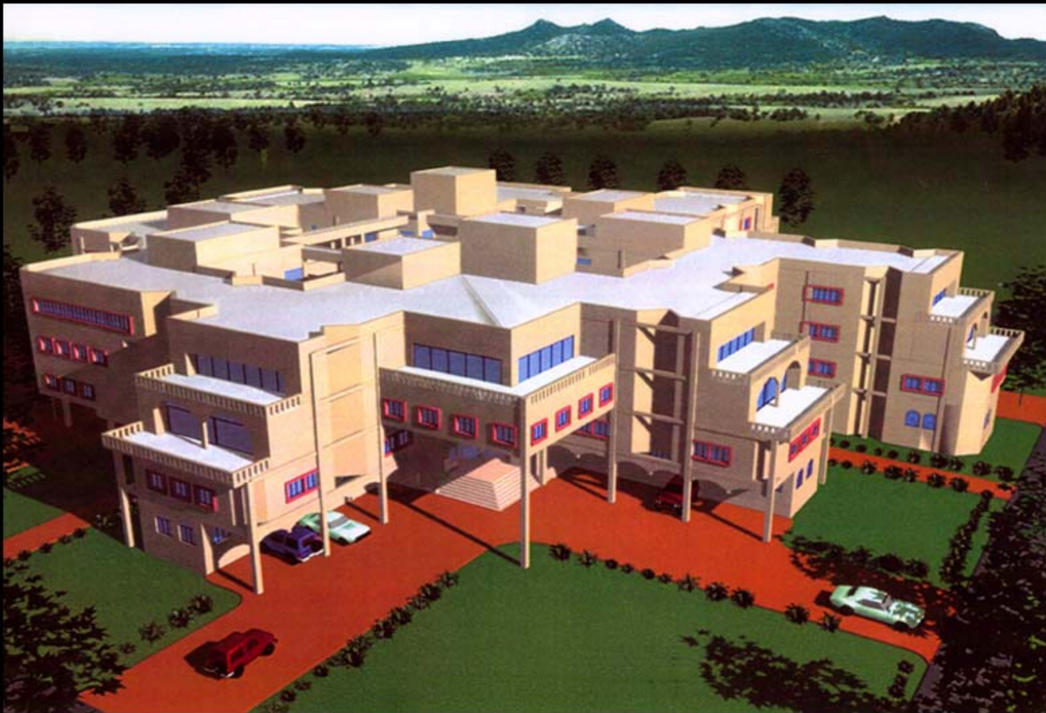
ADMINISTRATIVE BUILDING- ICD, DADRI
