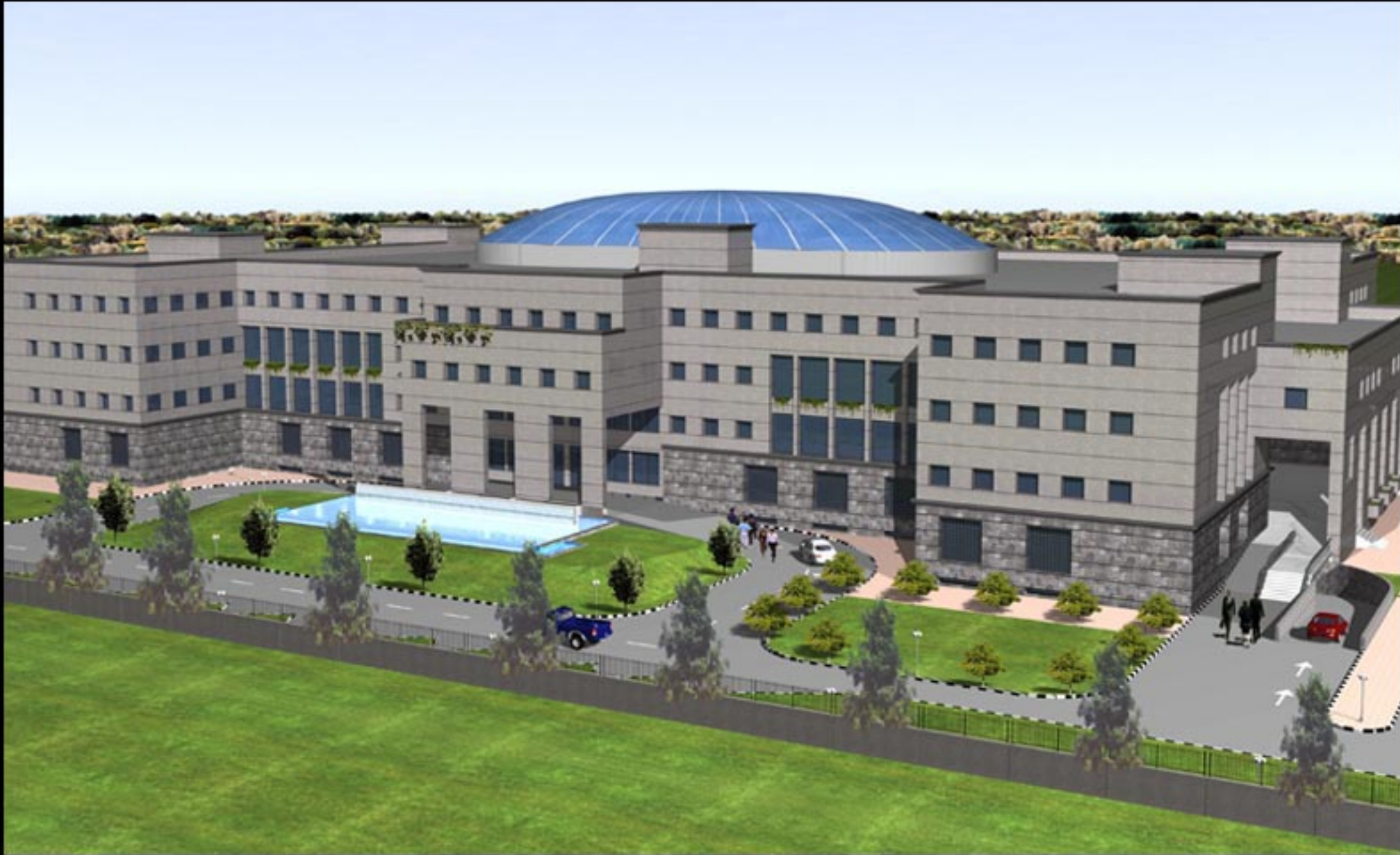
NATIONAL SOCIAL SECURITY REGISTRY AND PROCESSING CENTRE FOR EPFO AT DWARKA, DELHI
