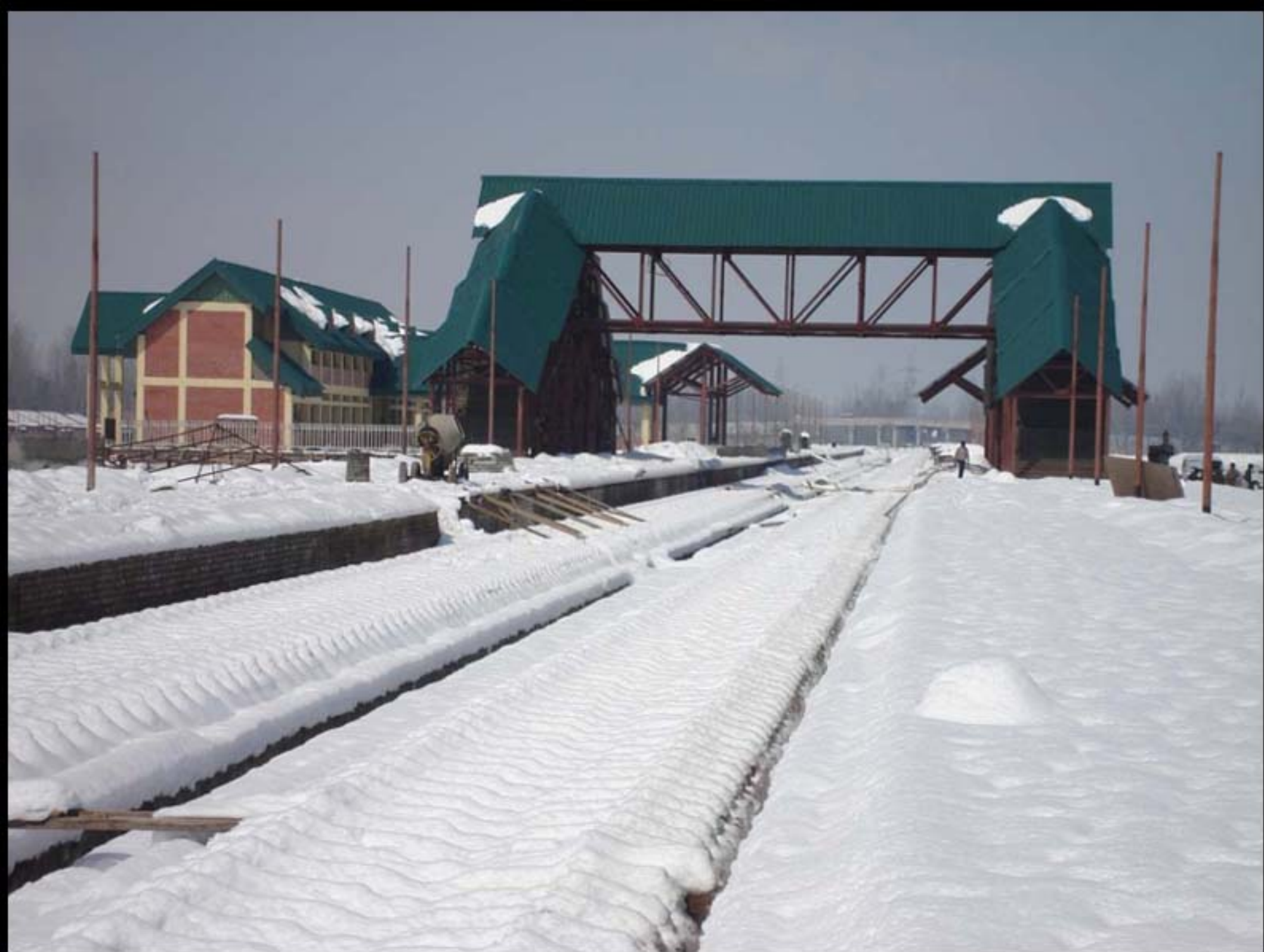
PAMPNORE STATION YARD
