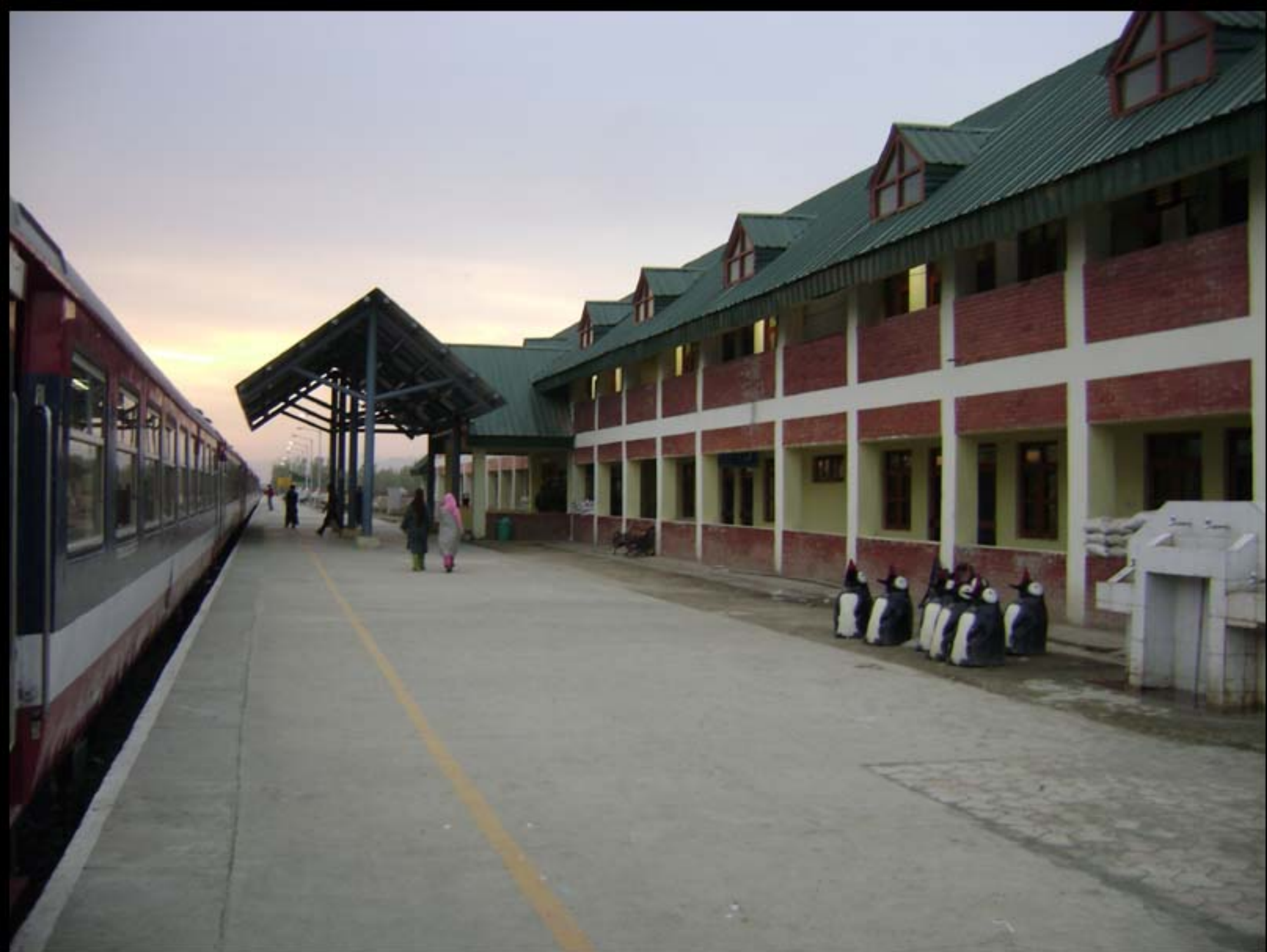
ANANTNAG STATION YARD
