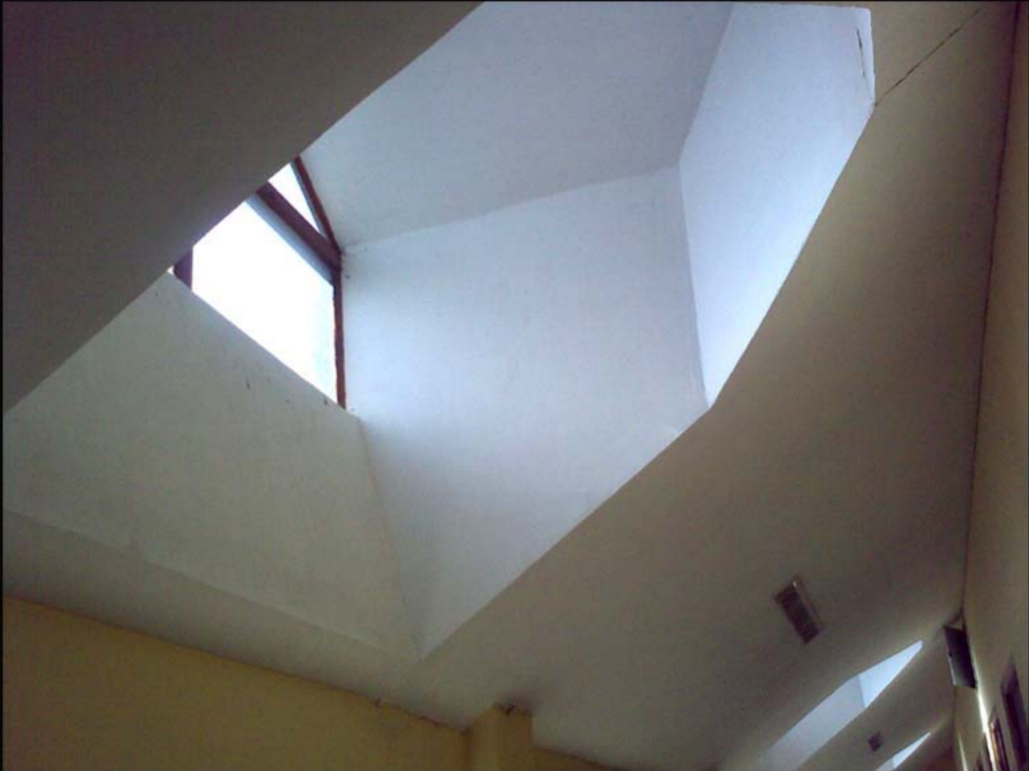
SERIES OF DORMER WINDOWS IN STATION AT ANANTNAG, J&K
