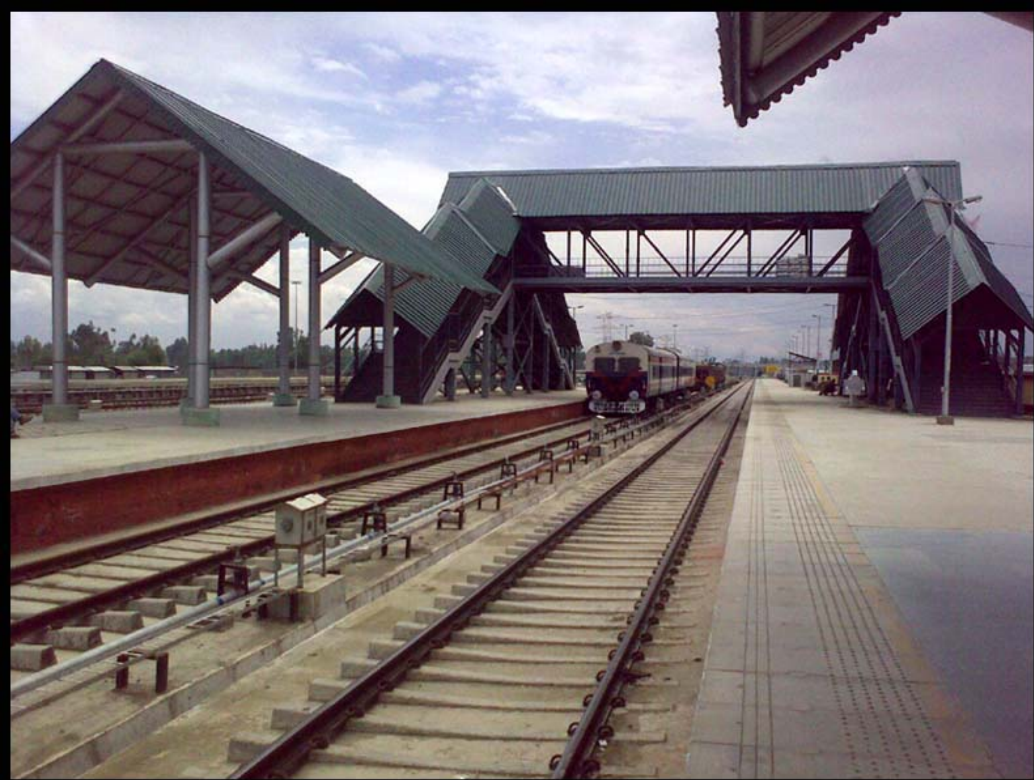
PLATFORM SHELTER & FOOT OVER BRIDGE AT BADGAM, J&K
