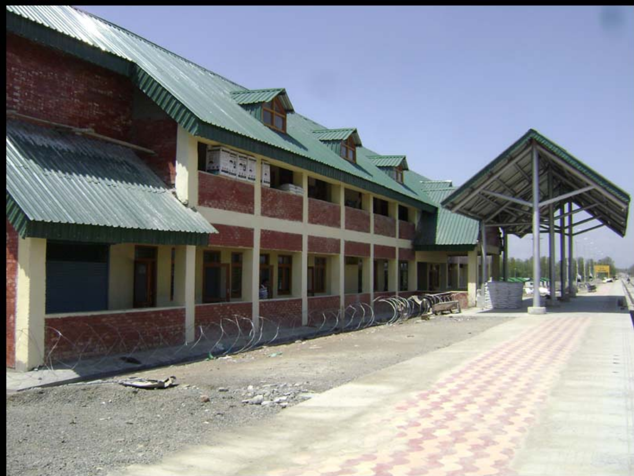
HAMRE STATION YARD
