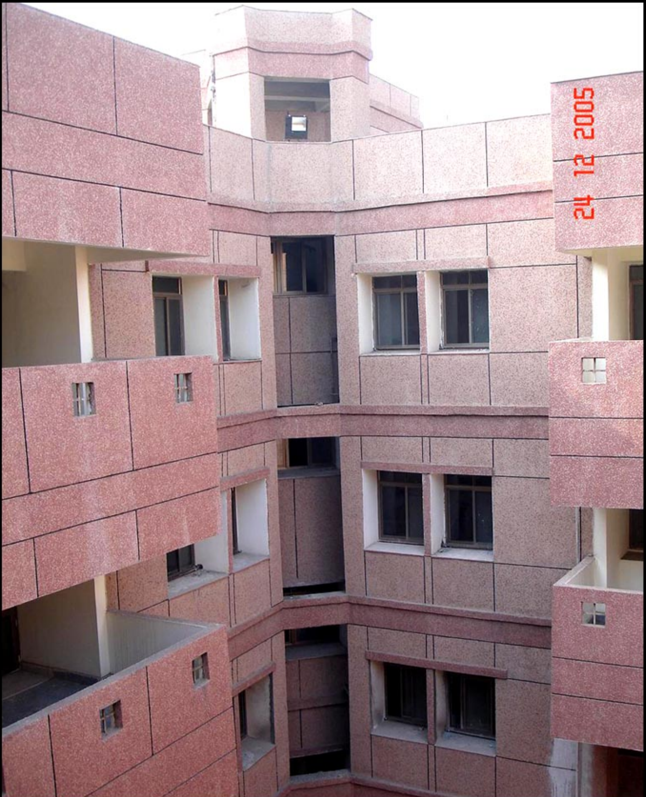
INTERNAL COURT OVERLOOKED BY BALCONIES, BHAGVAN MAHAVIR HOSPITAL, PITAMPURA, DELHI
